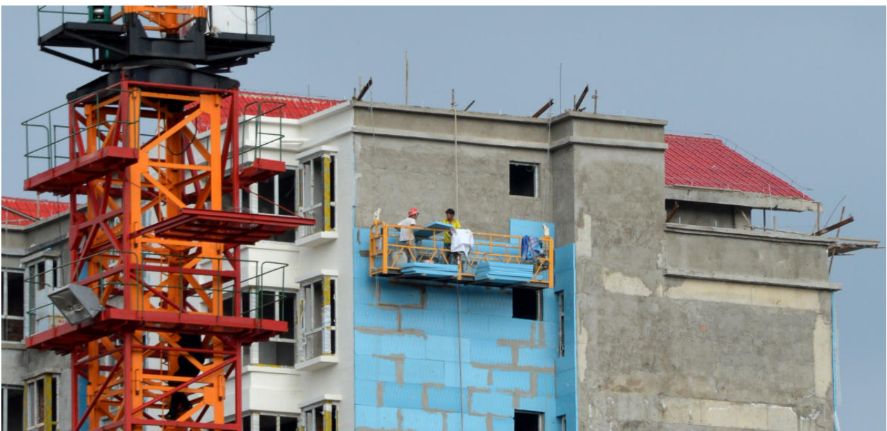
Figure 15: A residential building in Hezuo, Gansu province, is fitted with insulation panels.
