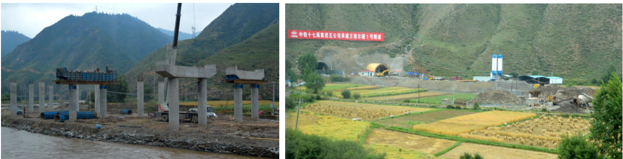
Figure 8: The highway from Linxia to Hezuo under construction.
