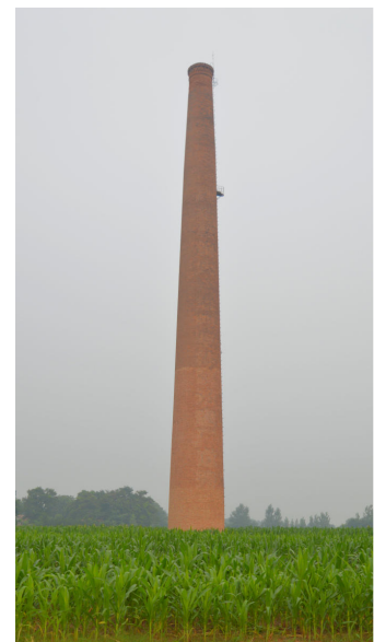
Figure 5: A lonely chimney in a corn field is all that is left from a brick factory in rural Henan province
